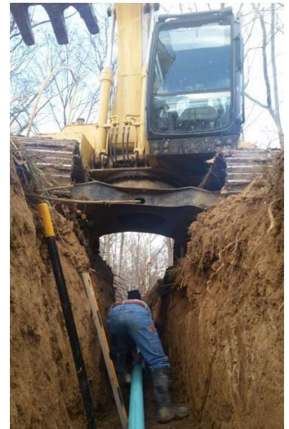
ASUC have provided the picture, right, showing the risks associated with working in deep excavations.
